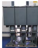
DSS A Merlin Gerin Ringmaster CE2 200A SF6 CB SE6 630A SF6 Switches
