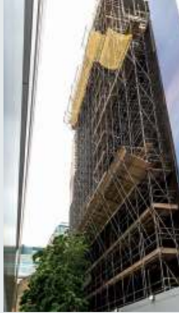
100 Liverpool Street part of a wider redevelopment of Broadgate
