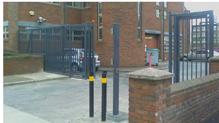
Wicket gate installed adjacent to a vehicle gate.
