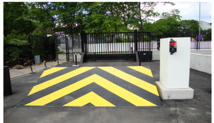
Terra Blockers control cabinet installed next to blocker
