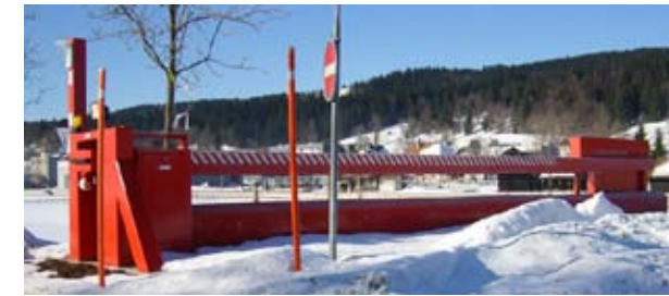
Team Beam whilst open
