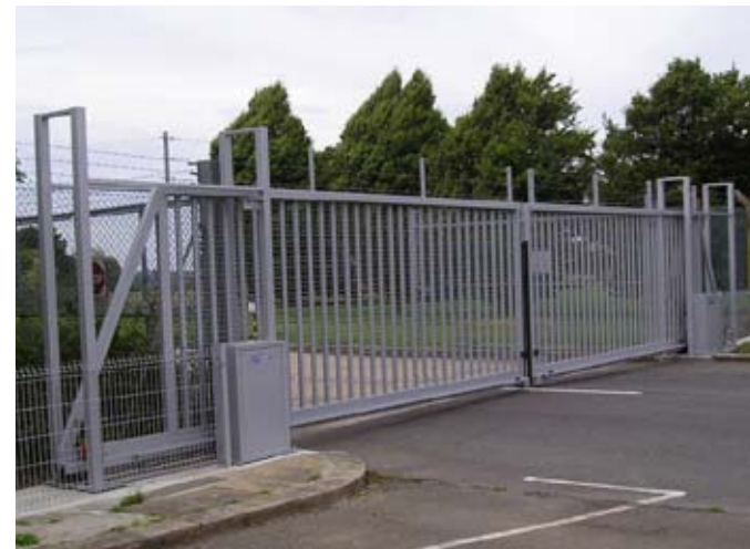
Bi-parting pair of Sliding Gates which can operate individually for smaller vehicles or together for larger vehicles.
