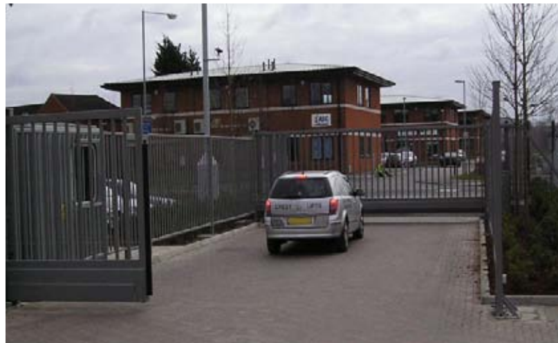
Sliding Gate interlock system
