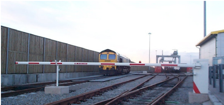
HB Barrier securing 10m aperture
