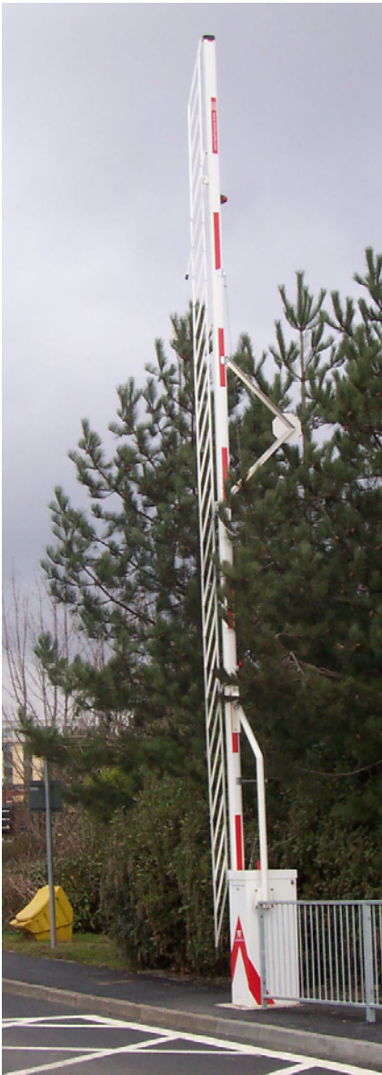
HB Barrier in the raised position.
