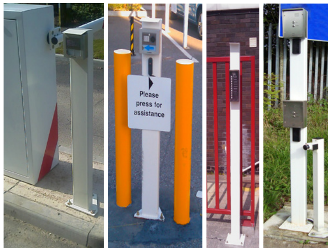
Standard Car Height Pedestals. Installed with bollards for protection
