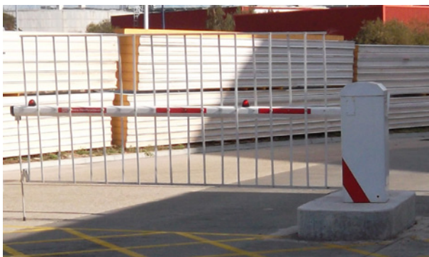
FB Barrier installation with typical base foundation
